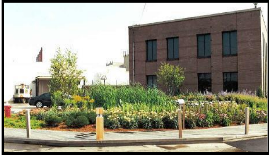
Figure 4: Subsurface Flow Wastewater Treatment Wetland at Saginaw Metal Castings
